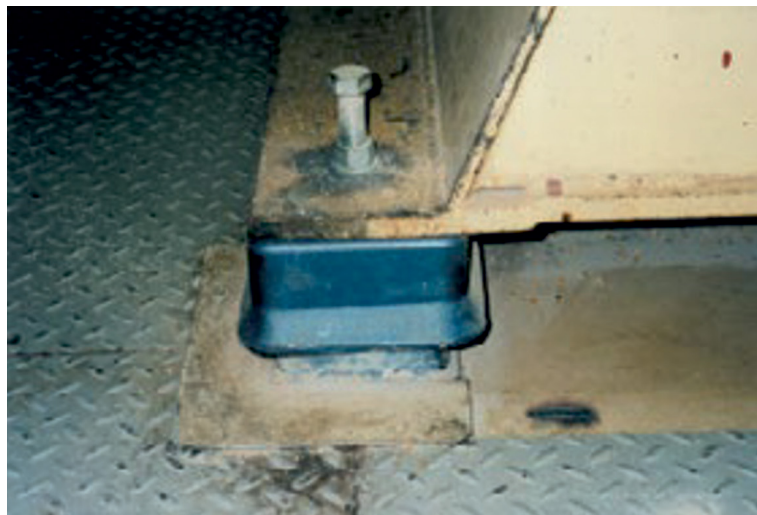
Figure 7 Detail of vibration-isolating mount
